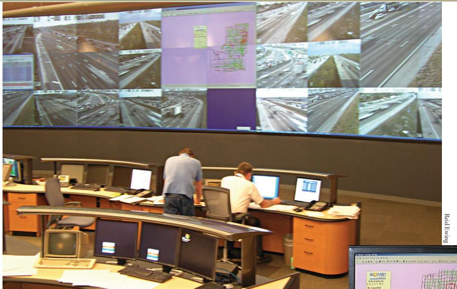
Broward County's High Tech Transportation Management Center. The map shows intersections on-line (green); communication failures (red); and the controller failures (purple).
