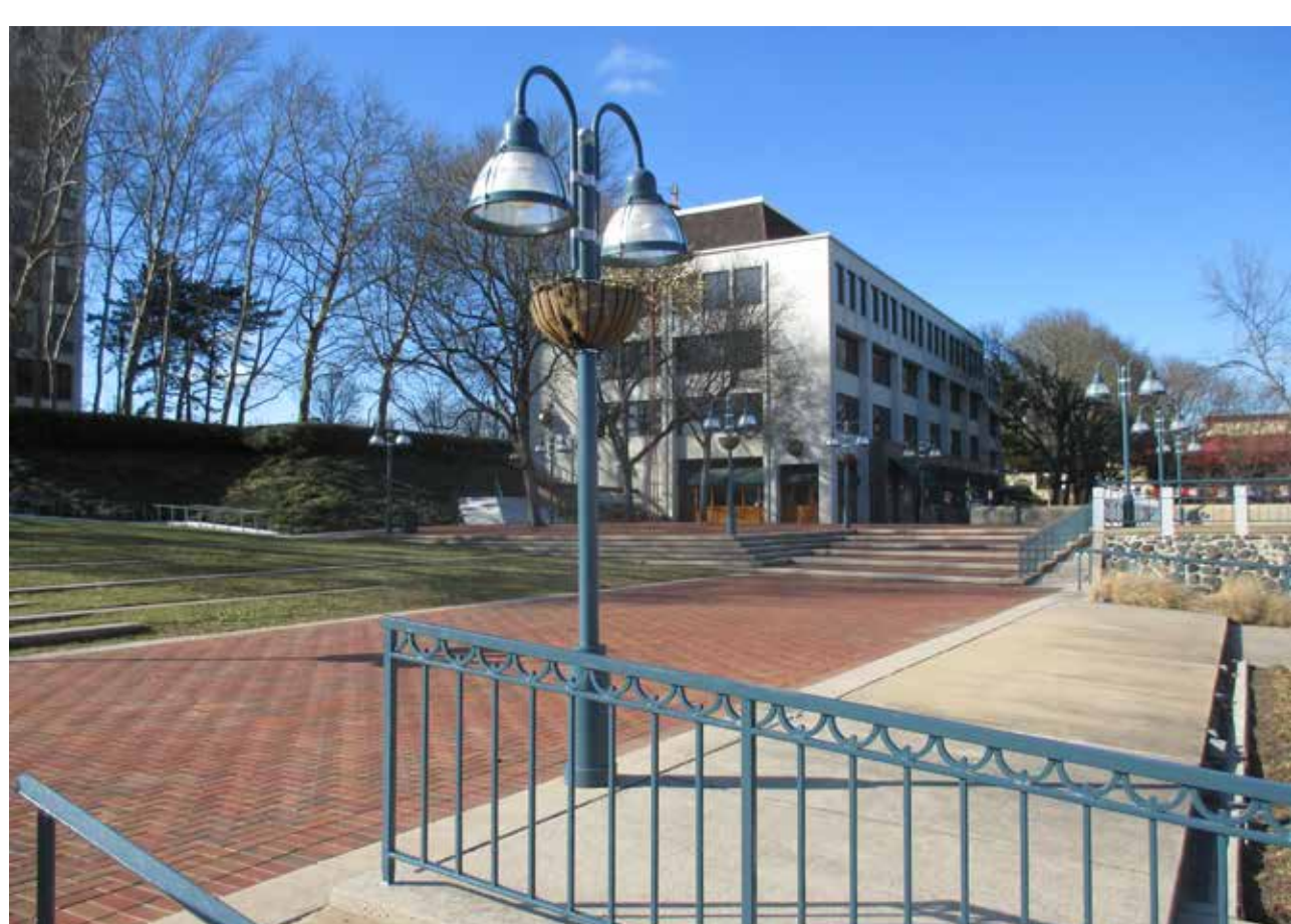
Outdated fixtures/railings do not match modernist style.
