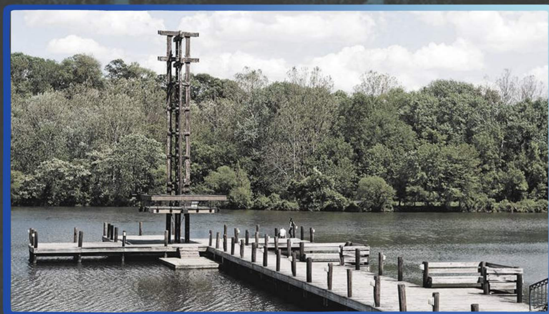
Before Bell Tower
