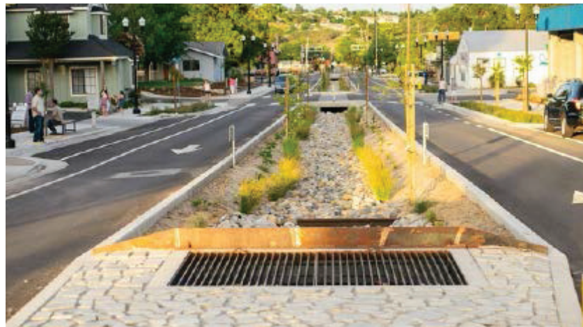
Adaptive reuse of railroad tracks as curbside rain garden: 21st Street Paso Robbles, CA http://www.svrdesign.com/21st-street-paso-robles-ca/
