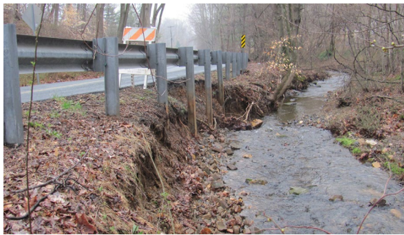
Figures 1 and 2: Examples of streambank erosion
