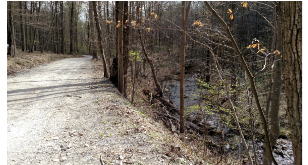
Figure 42: Roadway crossing stream.
