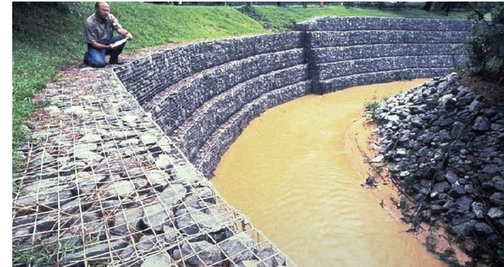
Figure 47: Gabion Wall for Steep Slope Protection
