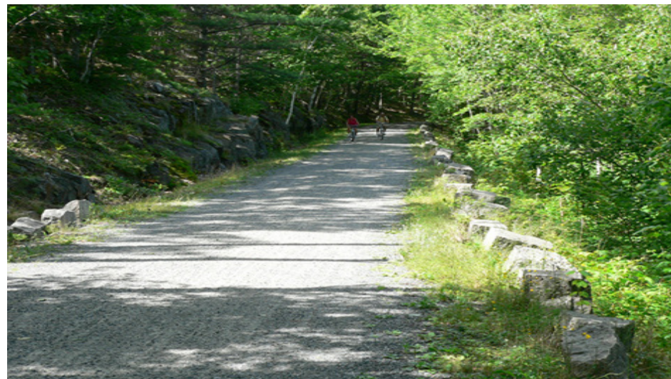
Figure 44: Boulder protection from roadside parking.
