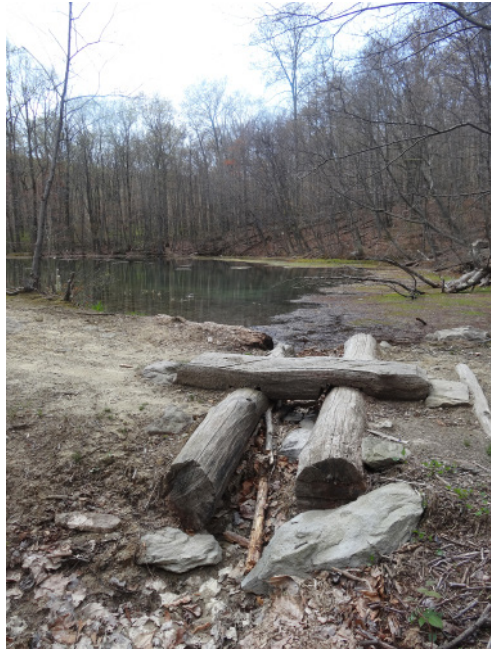
Figure 32. Pond outlet too small
