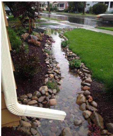
Figure 17. Disconnected downspout (Brown, 2019)
