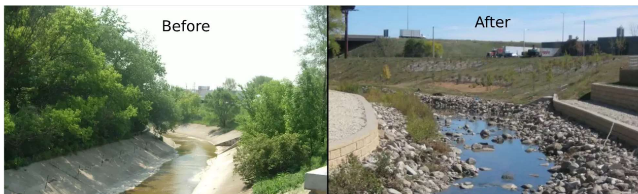
Figure 14. Stream restoration where hydrologic connectivity is restored (Maeder, 2019)
