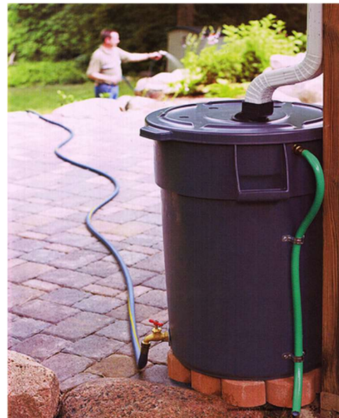
Figure 18. A garbage can used as a rain barrel (“Great DIY Rain Barrel”, 2011)
