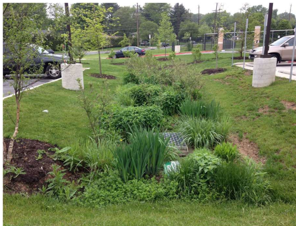
Figure 19. A rain garden (Montgomery County Government, 2019)
