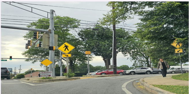
Channelized turn lanes like this one at Connecticut Ave and East-West Hwy enable drivers to make high speed turns and reduce pedestrian safety and comfort.
